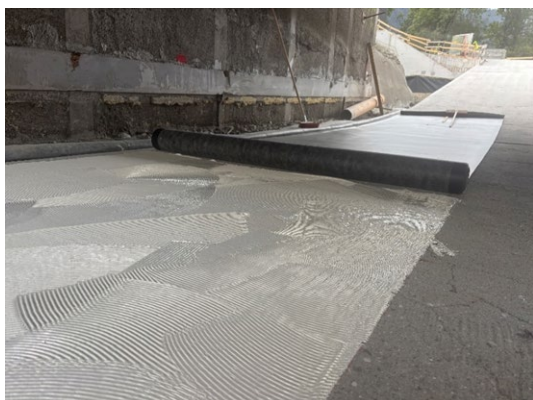
Fig. 6: Pose de SikaRoof® AT
