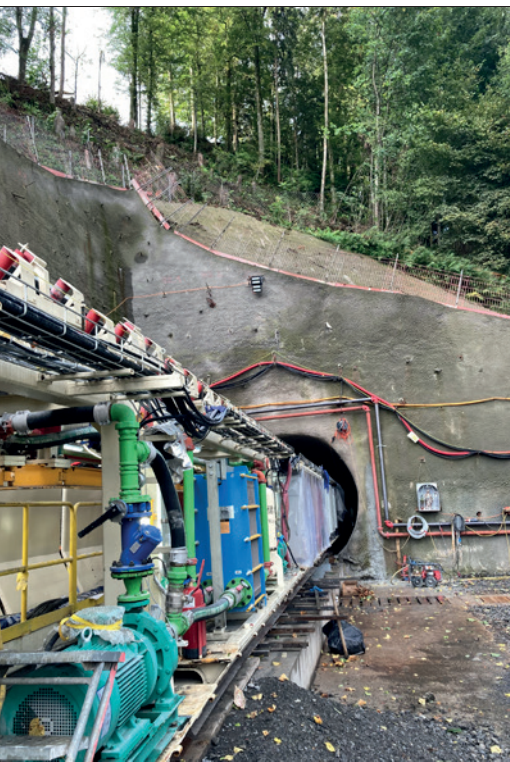
Tunnelbohrmaschine am Start.
