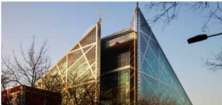
Park View Green Plaza, Beijing, 2010 Beratung ARUP Hong Kong; Fassade Beijing Jianli (CN)
