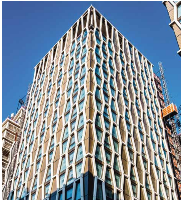
The Broadway London, 2021 Architekten Squire & Partner; Fassade Focchi Spa
