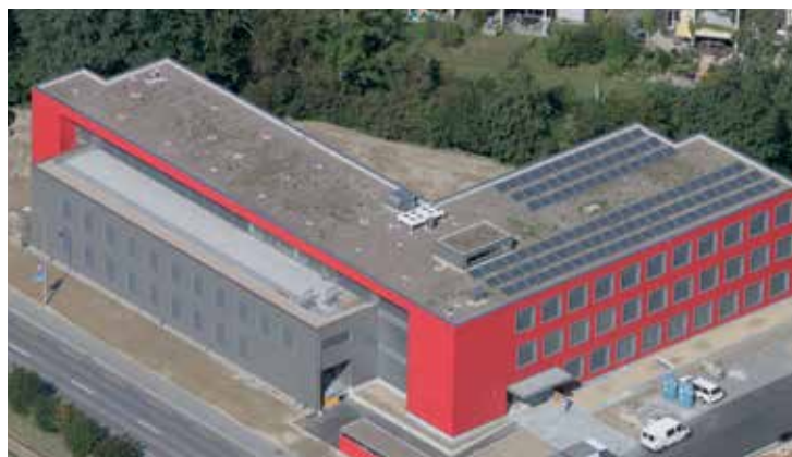
Station ornithologique Sempach: Minergie-PECO
